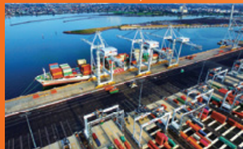
VICT won the award for "Smart Infrastructure Project" in recognition of its automation at the 2017 National Infrastructure Awards, and gained the highest possible rating of "Leading" for sustainability from the Infrastructure Sustainability Council of Australia (ISCA), in line with the vision to be among the world's greenest terminals.
